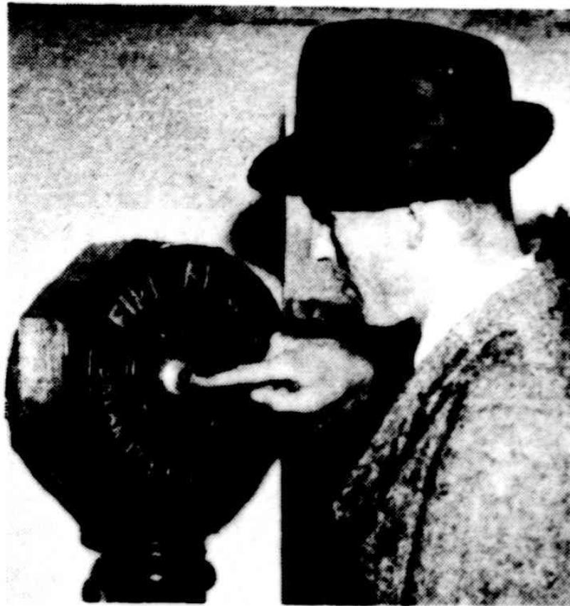
The new "Talkalarm" system to be installed throughout the city will enable the person detecting a fire to speak to brigade headquarters after pressing the button shown here.
